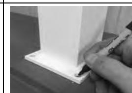
3. Remount the post assembly. Insert the appropriate fasteners then secure the base to the deck structure. Make certain the posts are plumb. If the post requires adjustment, add stainless steel washers under the base plate. Do not re-install the base post trim until step 2 of the rail installation.
