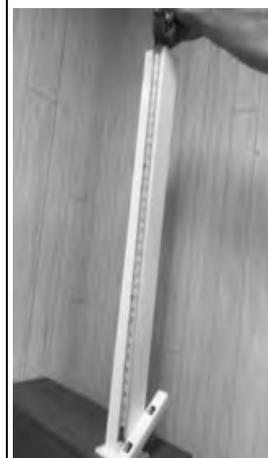
2. When the final position is determined for the post, mark the hole locations of the four 3/8" diameter mounting holes provided on the base and remove the post assembly. Drill the marked locations into the decking and reinforcement using the proper size drill required for the fasteners being used.
