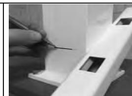
2. Install the base post trim on both the upper and lower posts.
