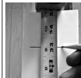
4. To locate the mounting hole locations of Top Rail Hinge Assembly (C) and the Bottom Rail Hinge Assembly (D) place a mark 1" above and below each of the level line marks centered on the posts from step 3 (see photo) This will be the location of the fasteners to attach the Hinge Assemblies to the post.
