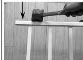
*Note: Notches are provided on the front of the box to help align balusters and aid in the assembly of the rail in this step.*
